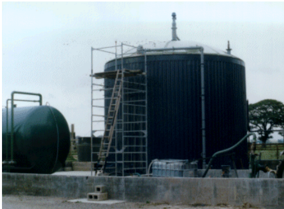
Anaerobic Digester-Farm Size
